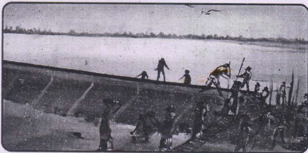
Almost completed of construction of Barrage
