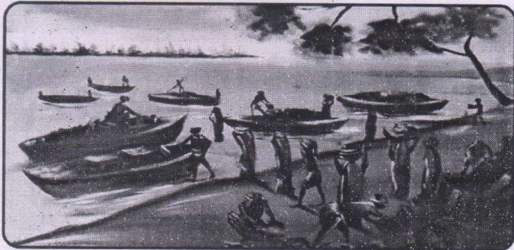
Carrying the stone slates in local country boats for construction of Dam.
